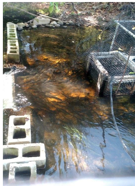
Spent alewives leaving Bride Lake. The upstream counter and trap are detached to allow this emigration. Spent alewives depart in large numbers all at once and we have to open the spillway to avoid mass mortalities.
