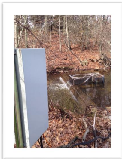
The Bride Brook fish counter is installed but the trap is not yet in. Fish swim over the little weir and pass through the counting array and data are recorded in the silver lock box in the foreground. The trap, which will allow us to capture fish and truck them to other watersheds, will be installed soon.
